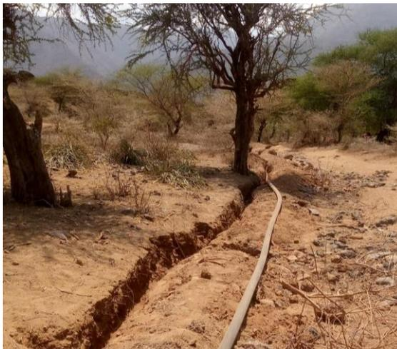
*2-inch HDPE plastic pipe in trenches after steel pipe*
