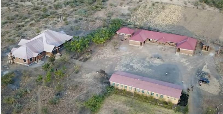
Drone photo of Engaruka English Medium Primary School. Crane Classroom and Restroom Buildings upper right. Peter Ozolins Dining Hall left. TX Foundation Pre-school Building lower right.
