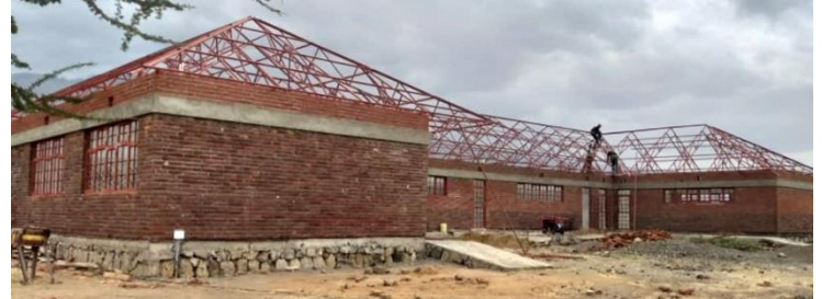
Crane Classroom and Library Building construction. July 17, 2019.
