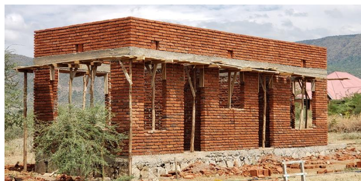
Powerhouse June 12, 2019. Windows, doors and roof installed in July.
