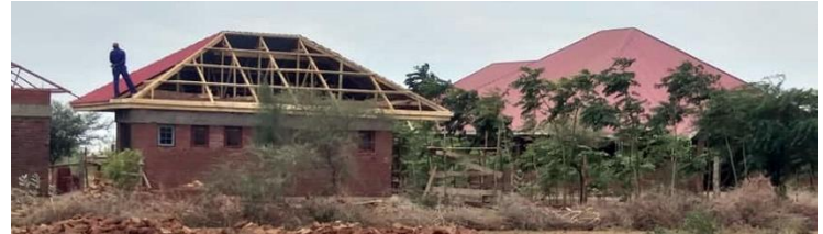
New restroom building. Dining hall behind trees. July 17, 2019.
